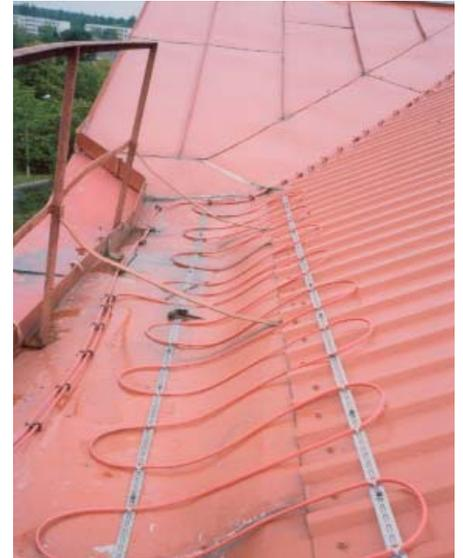
cable from mechanical damage, direct sunrays, and fallen leaves, seeds etc.
