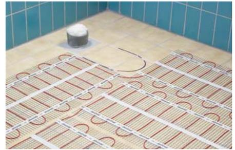
The installation of the devimat™ should be started from the wall and directed towards the opposite wall. Here, the mat needs to be turned back by cutting the net of the devimat™ (NB! DO NOT cut the cable!). This process has to be continued until the entire surface has been covered with the devimat™.
