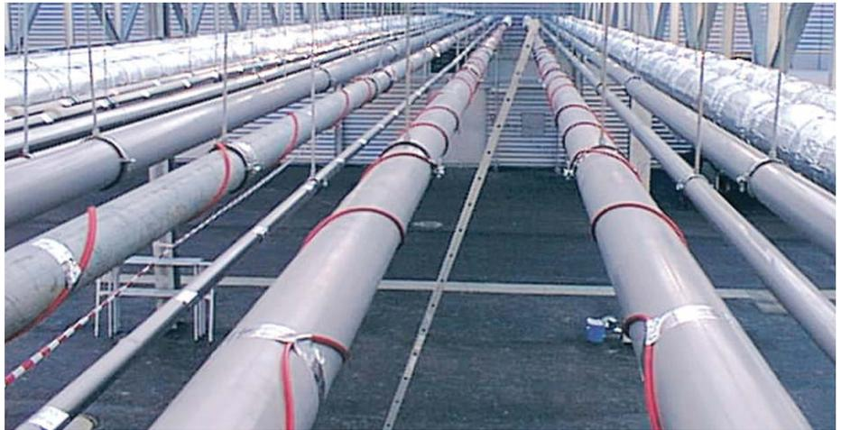
DEVI's pipe tracing systems may be used on the inside and outside of pipes, for indoor and outdoor pipe networks as well as for pipes above and below the ground.
