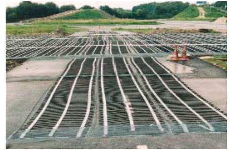
is not necessary to cover the cable with sand. This reduces the time and installation costs. In order not to damage the cables, heavy machinery (rollers or asphalt laying machines) should not be used on the cables.
