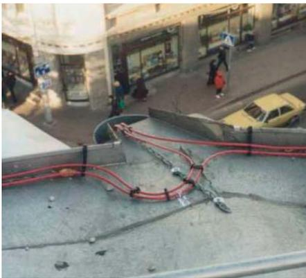
The heating cables can be installed in different ways in roof gutters and downpipes but in most cases the same cable is used for both roof gutters and downpipes.
