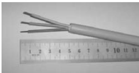
5. Remove the outmost 50 mm of the secondary insulation, too. Now, strip off approx. 10 mm of each of the three conductors.
