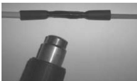
14. Crimp tube 12/3, L=150 mm is pulled over the entire connection. The crimp tube is crimped down from the middle out towards the ends.
