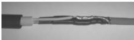
13. The heating cable screen is connected with the  $2.5 \text{ mm}^2$  rivet on the cold tail screen/ground wire. The rivet is squeezed onto it.
