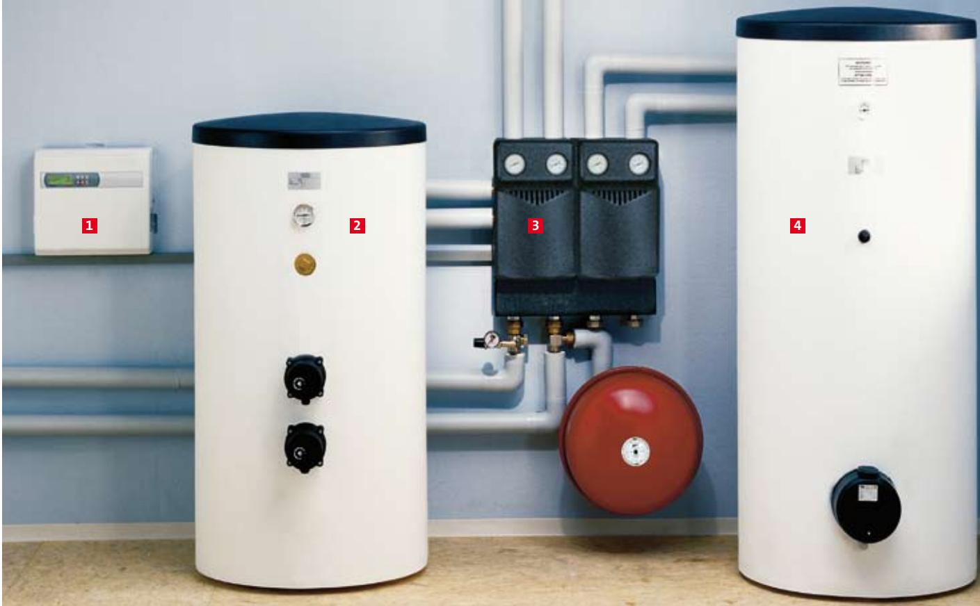
1 Heat pump manager 2 Buffer tank 3 Distribution system 4 Hot water cylinder
